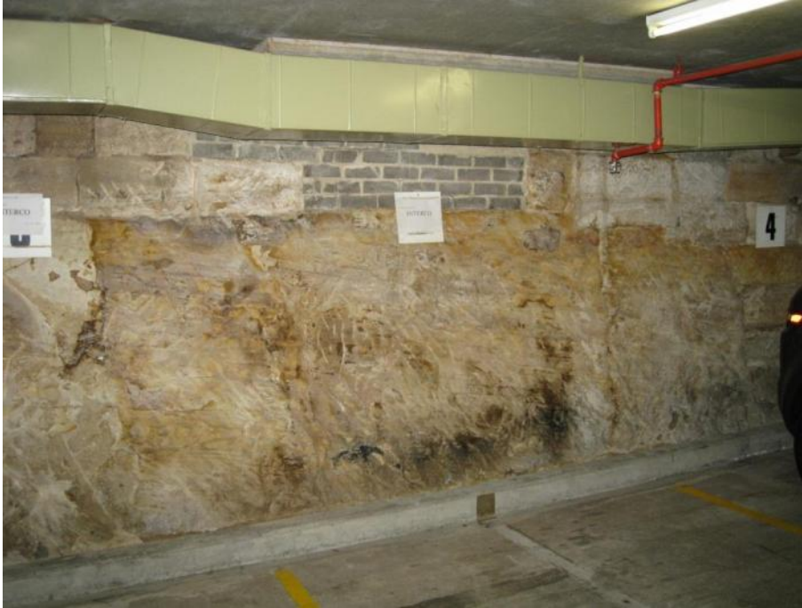
Figure 8 Exposed sandstone of 2-10 Loftus Street
